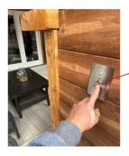
Step 3) Press the IGNITOR button on the right of the fireplace. You will hear clicking that will ignite the gas
