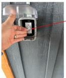
Step 2) Turn the timer switch past the 2 HOUR mark
